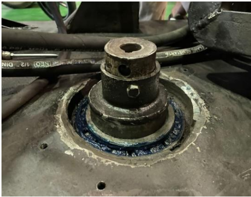
Gambar 12 Pemasangan stopper taper bearing
