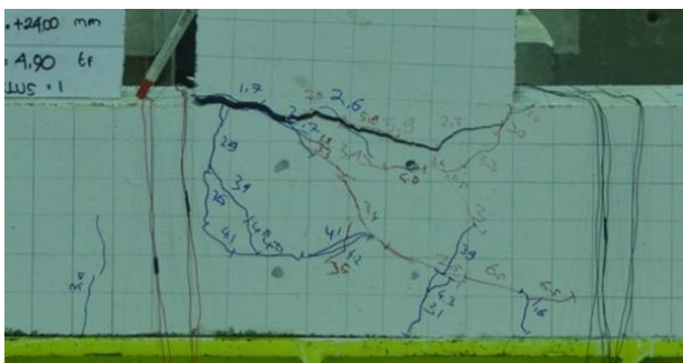
Figure 8. Crack Pattern of the Tensile Load (+), 24 mm
