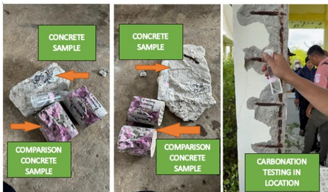
Figure 6 Results of carbonation testing on concrete debris and structural elements
