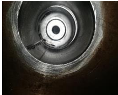
Figure 4. Holes After Alignment Process
