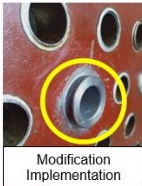
Figure 9. Implementation of Modifications on Oil Cooler GT PLTU Labuan
