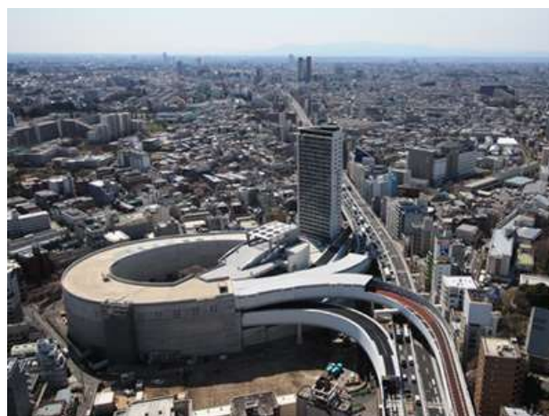
Figure 7. A bird's-eye view of a junction connecting viaduct with underground expressway in Tokyo (Metropolitan Expressway Company Limited. HP, 2011)
