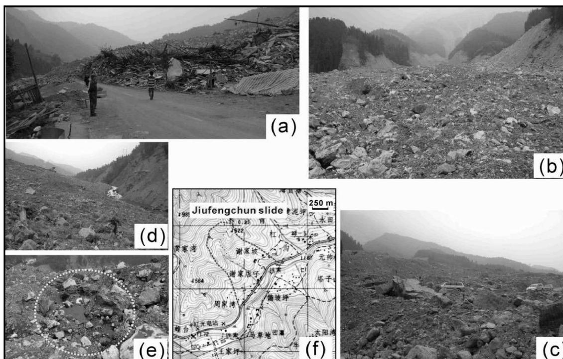
Figure 2: The rock sliding-rock flow in Jiufeng-cun Village. (a) Toe part, (b) Flowing path, (c) Oblique view, (d) Dammed river, (e) water in the sliding mass, (f) Old map showing a valley located along the flowing path
