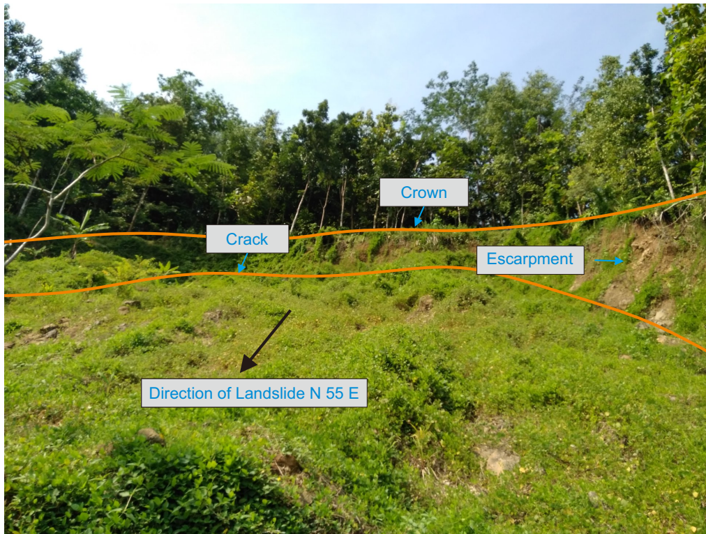
Figure 3. Landslide morphology on study area, Dusun Caok, Karang Rejo.
