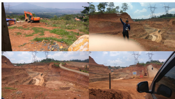
Figure 1. Cisumdawu Toll Road Construction
