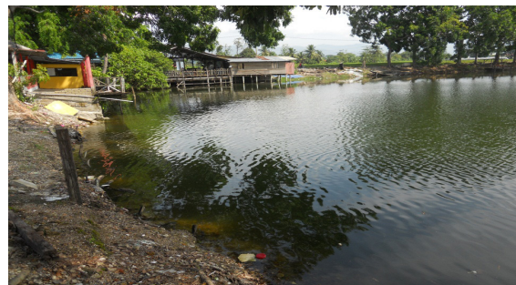
Photo 1. Restaurants that are located near lake Kg. Temiang which channel their domestic water waste directly into the lake
